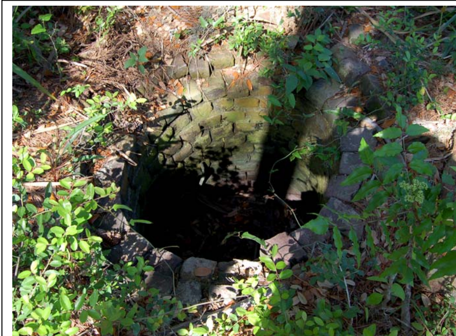
Figure 56. View of the well at 38CH1545.
