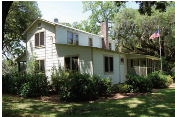
Figure 87. View of the structure located on the Mullet Hall property.
