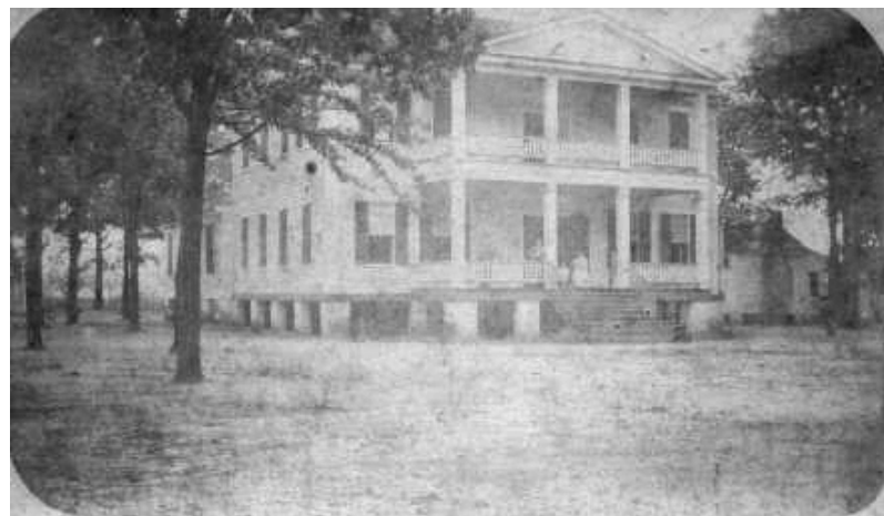
Figure 26. View of 38CR133 showing different yard features and a side structure.
