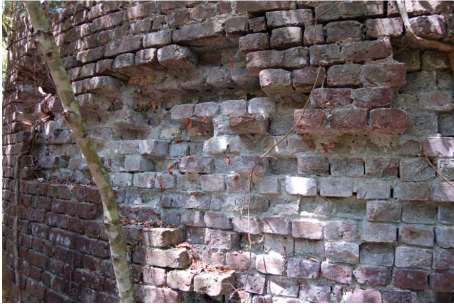
Figure 22. View of missing brick from the storm shelter.
