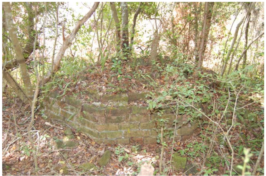
Figure 30. View of the octagonal chimney base at 38CH2114.
