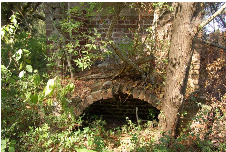
Figure 27. View of an arched hearth at a chimney in 38CH2113.
