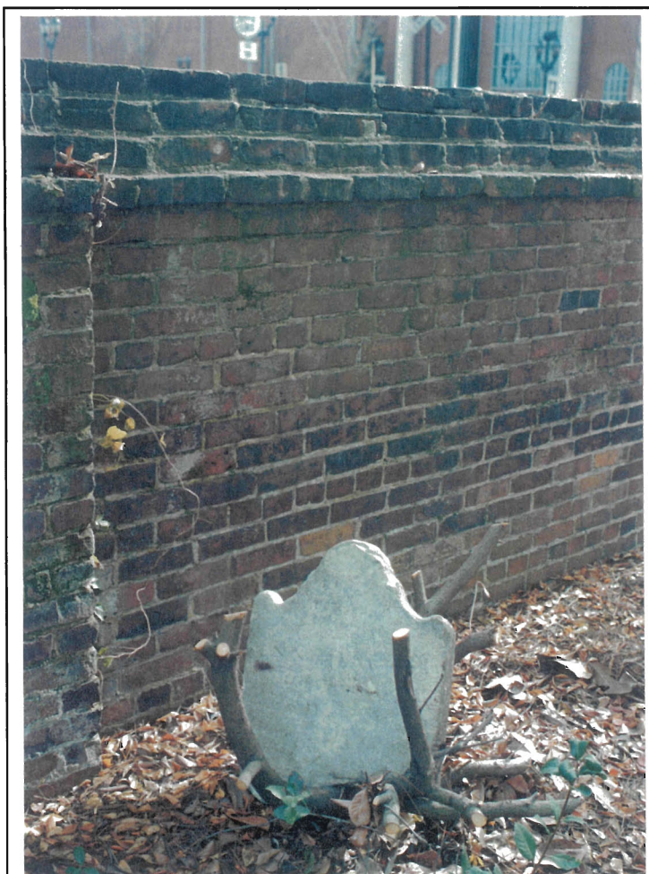
Figure 5. Loose stone found cradled in pruned bush, suggesting it may have been dropped there by an individual scaling the wall.
