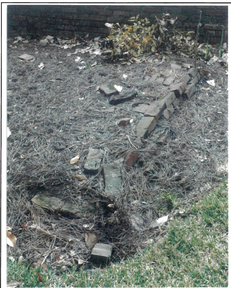
Figure 34. Probable hogback brick vault at St. John's. Additional investigation is necessary to determine whether enough of this vault has survived to allow reconstruction.
