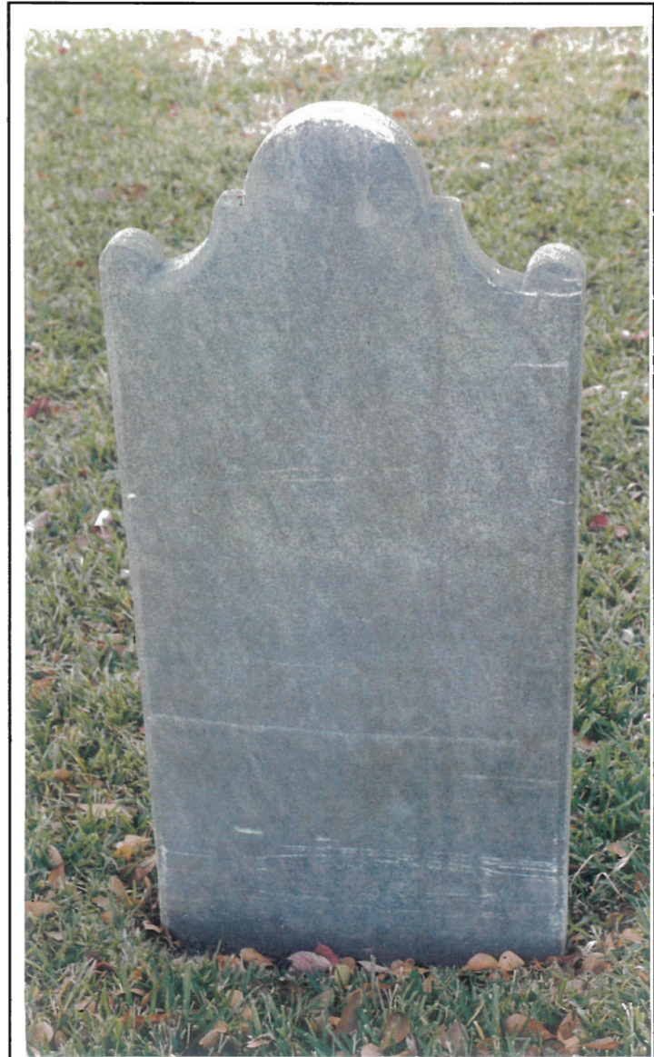
Figure 6. Reverse of a marble tabletstone showing mower and nylon trimmer damage. The striations on the upper two-thirds are likely from riding mower damage. The numerous parallel striations at the base are from nylon string trimmers.
