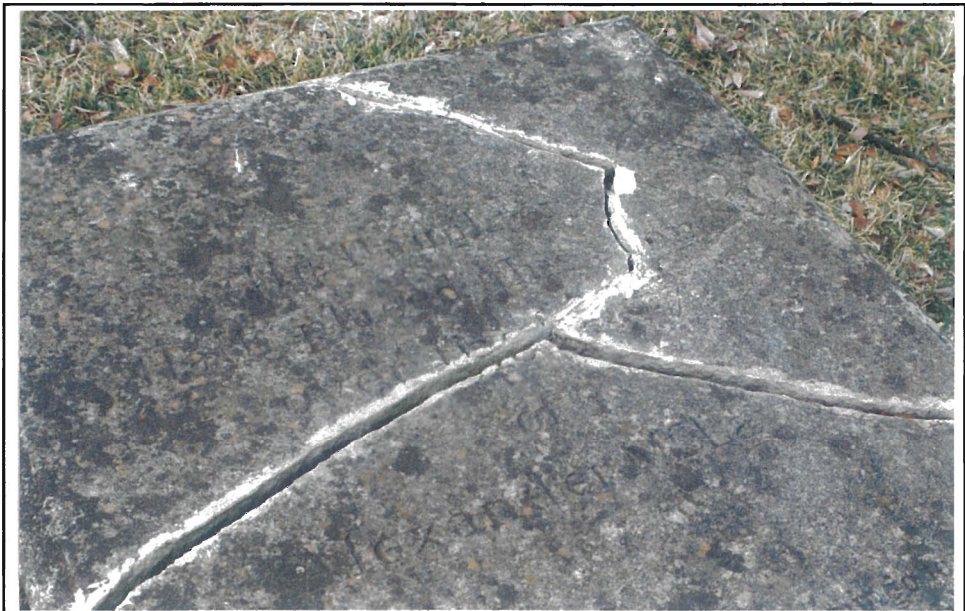
Figure 29. Example of broken ledger (Alexander McLaws) with failed previous repair. This stone requires mechanical repair before it suffers additional damage.
