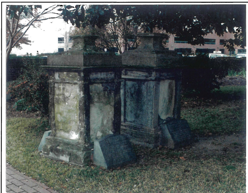
Figure 22. The installation of granite plaque markers on both sides of the Phinizy monuments makes it appear that they have "bumpers." Flush markers would have been far more appropriate and in keeping with the cemetery.
