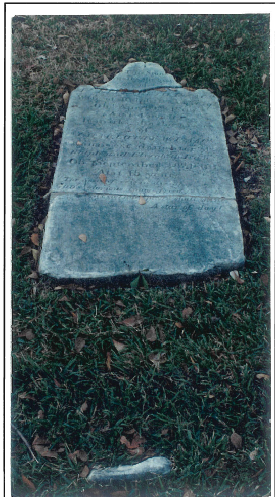
Figure 31. Broken tabletstone (Elizabeth & Charlotte Issacs) which needs to be repaired and reset with additional support. The footstone also needs to be reset.
