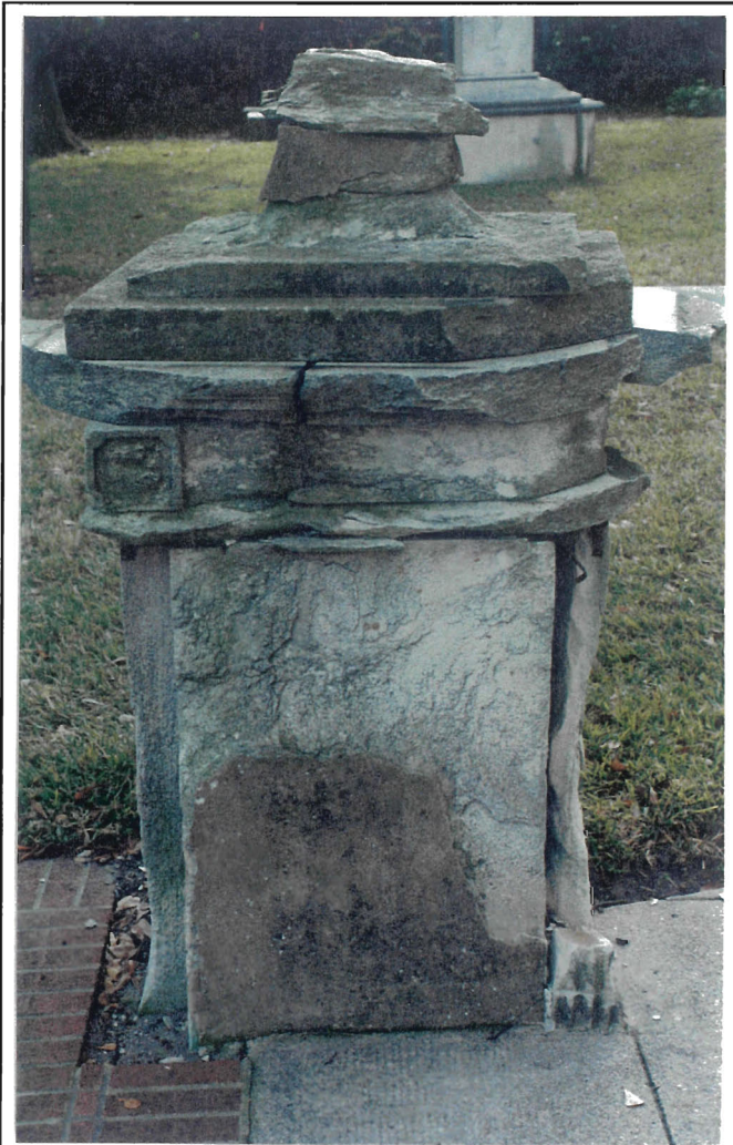
Figure 37. Example of severely delaminating schist monument at the entrance to St. John's. A previous effort to retard erosion is evidenced by the concrete patch on the lower half of the base. Most has already spalled off.
