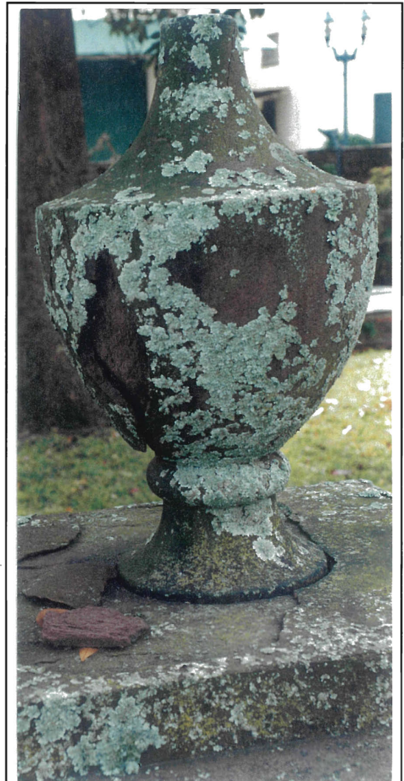
Figure 36. Contour scaling on carved urn topping the monument shown in Figure 35.
