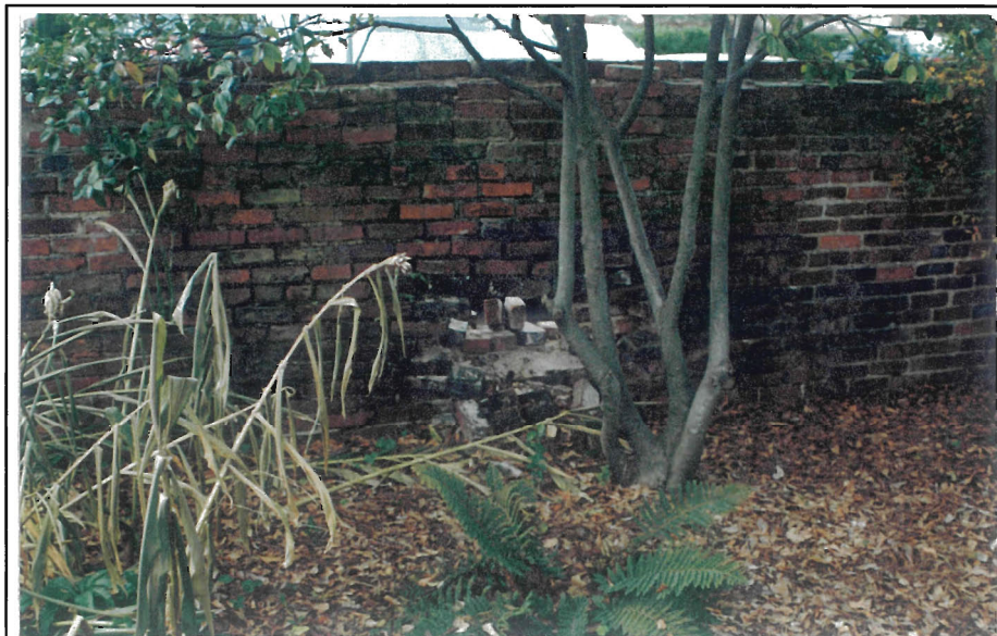
Figure 23. Interior damage to wall bordering the parking lot.
