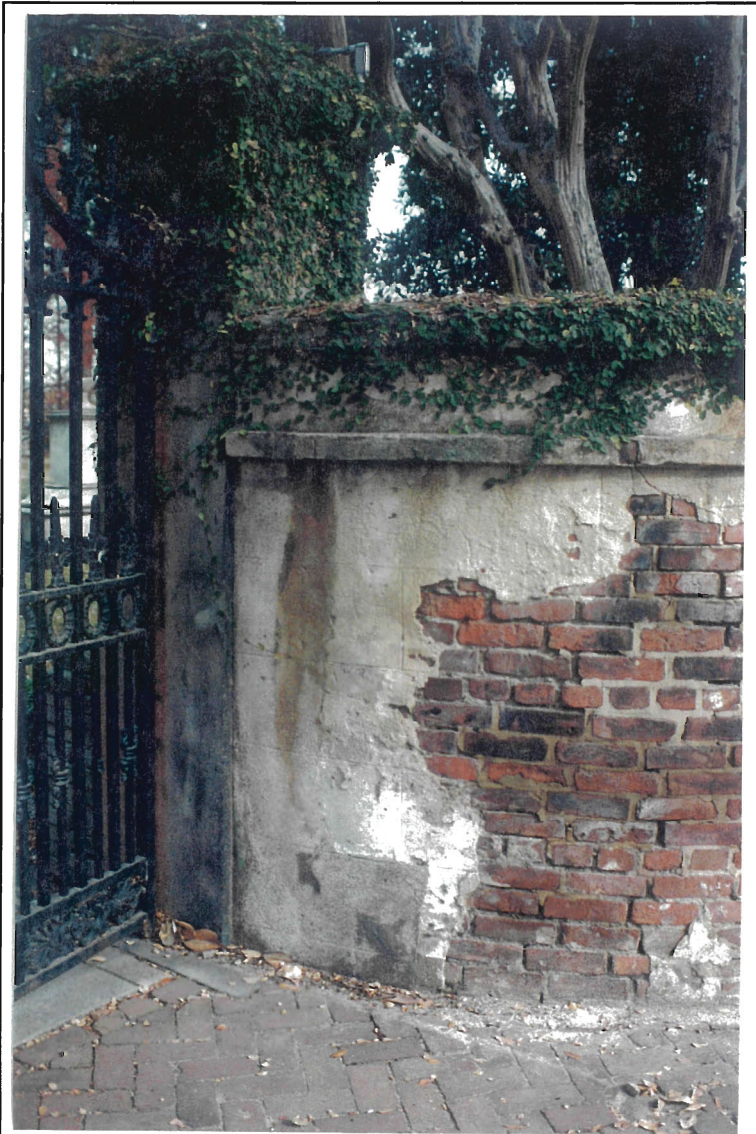
Figure 26. Example of deteriorated stucco at entrance. Here the vines need to be removed, the stucco documented, and then replaced with a product such as Jahn M60.
