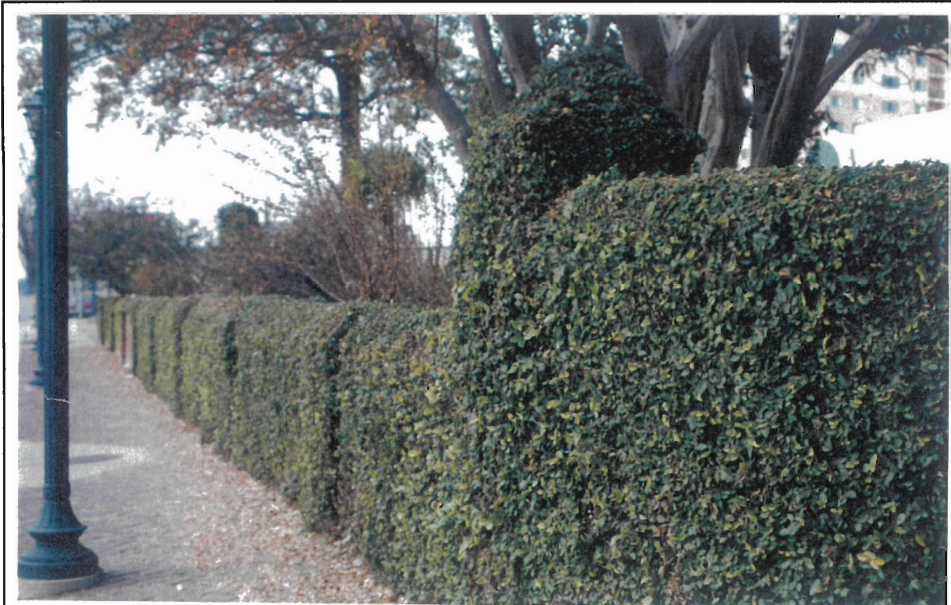
Figure 9. Vines attached to the brick wall along Reynolds Street should be removed to protect the stability of the brickwork.
