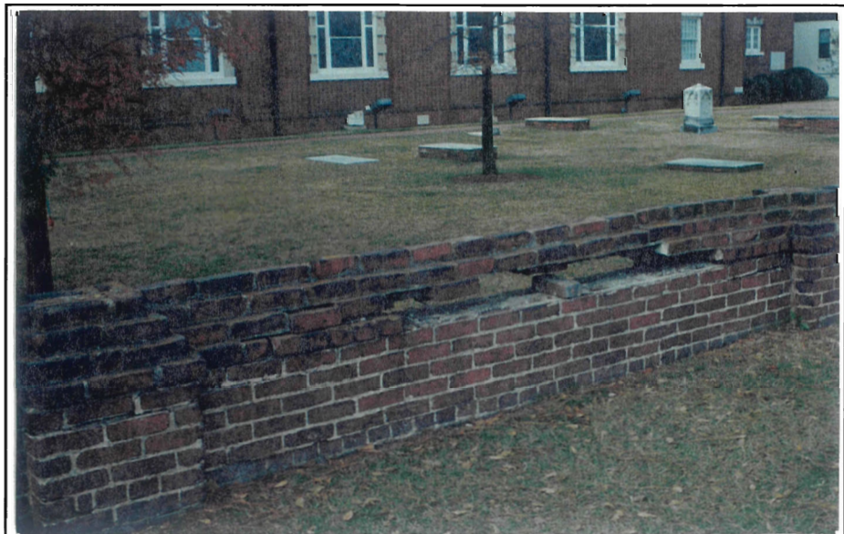
Figure 25. Damaged wall section along Sixth Street. About 25 feet of the top four to five courses will need to be disassembled and reset.
