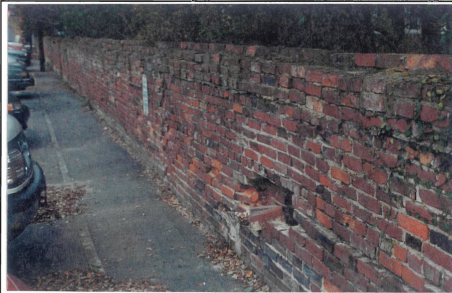
Figure 24. Damage on the parking lot side of the brick wall section shown in Figure 23. Note that the wall is bowed inward for a distance about 20 feet. All of this will need to be taken down and reset. There is no "simple fix" for this impact damage.
