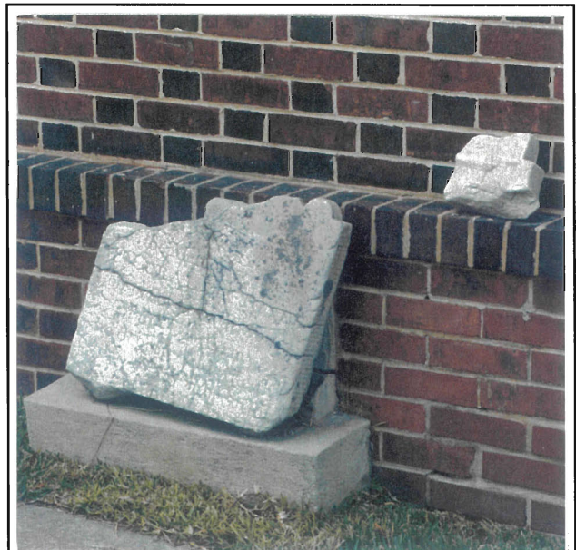
Figure 20. Broken markers leaning up against Church wall.
