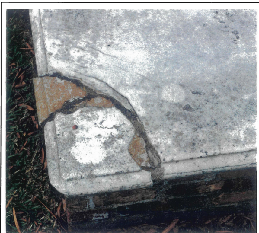
Figure 32. Example of an inappropriate, poorly executed repair. It is, however, stable and should be left alone until such time as it fails.
