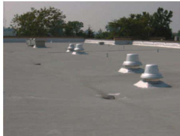
Roof traffic should be kept to a minimum and where expected, extra protection – such as walkway pads or roof pavers – should be provided. The roof inspection should also result in a written report that is kept on file.
