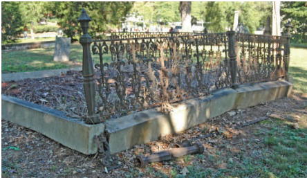
These before and after photos show the extraordinary difference appropriate repair techniques can make.
