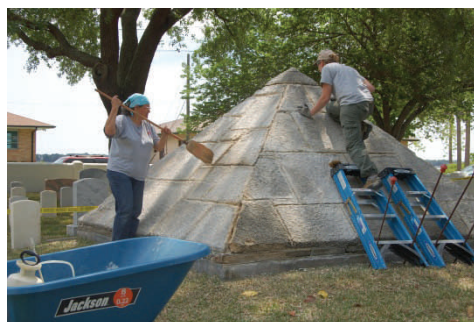
The hard mortar was cut out in preparation of repointing using a soft lime putty mortar.
