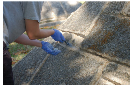
Lime putty being placed in the cleaned joints.
