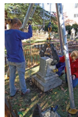
Chicora's team is carefully resetting a Trinity monument using a 1-ton tripod and lifting device.
