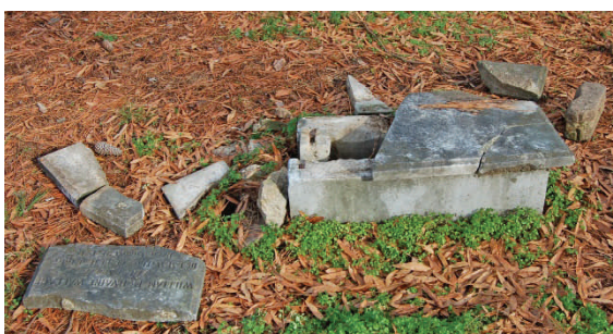
William McIlvaine Wallace Box Tomb before repair showing damage.
