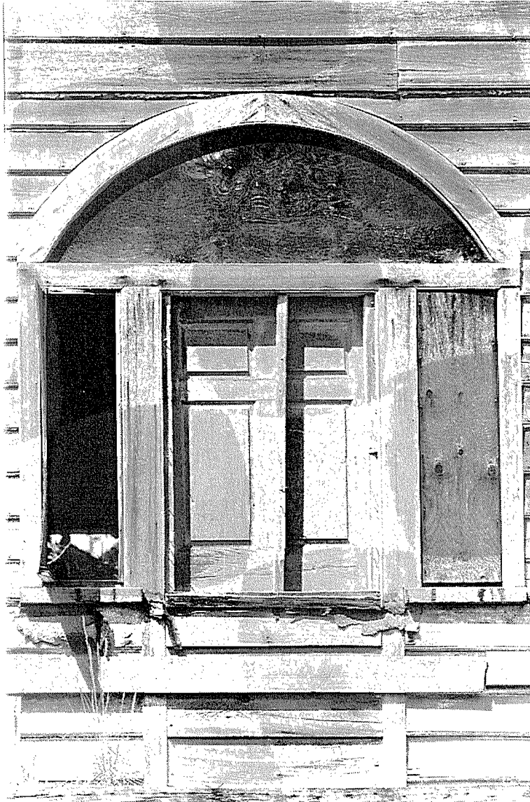
Figure 89. Stylistic elements surrounding the south second floor doorway.
