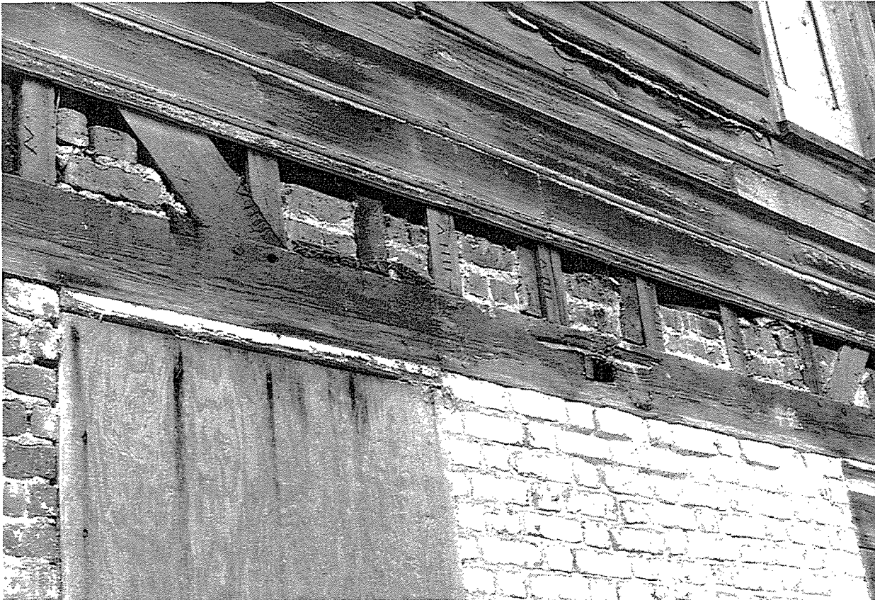
Figure 88. Carpenter identification marks on south facade framing.
