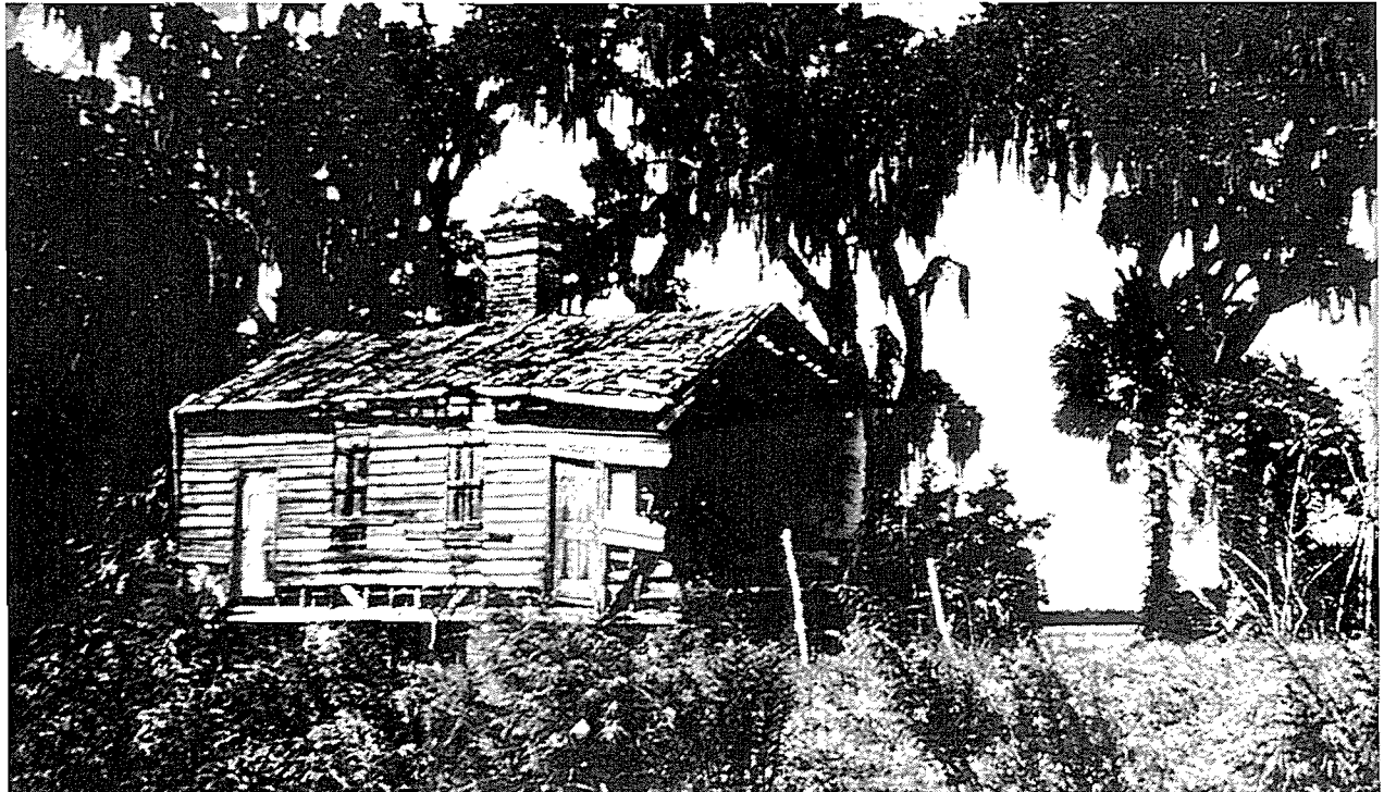
Figure 26. Vanderhorst kitchen, ca. 1945, view taken to the northwest (photo courtesy of Historic Charleston Foundation, Inc.).
