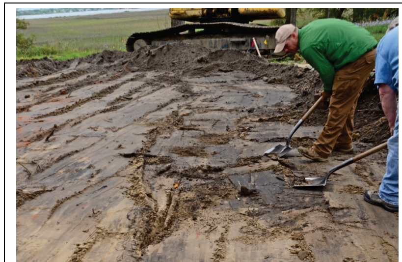
Figure 79. Shovel skimming feature during stripping operations.
