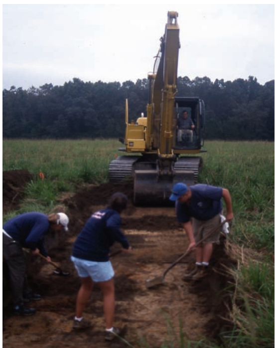
Figure 25. Track hoe excavating in the garden area.
