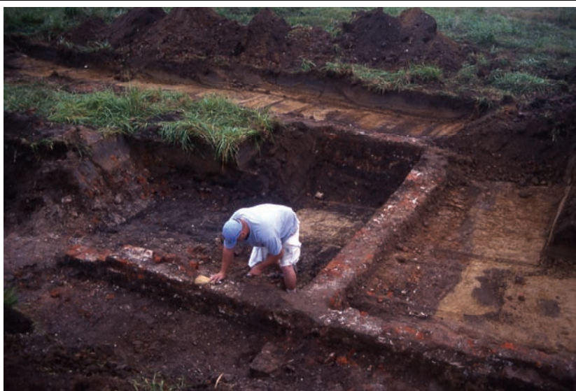
Figure 49. Cleaning one of the basement rooms with a brick floor. View to the northeast.
