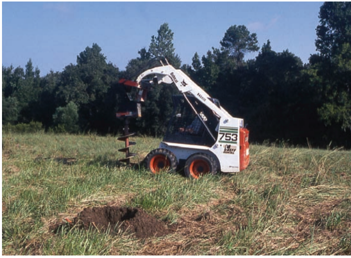
Figure 23. Auger testing with 18-inch power auger.
