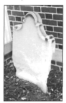
Severe efflorescence with stone loss.
