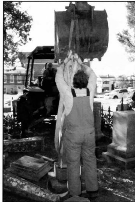
Straps are attached to the backhoe bucket using a 1" shackle.
