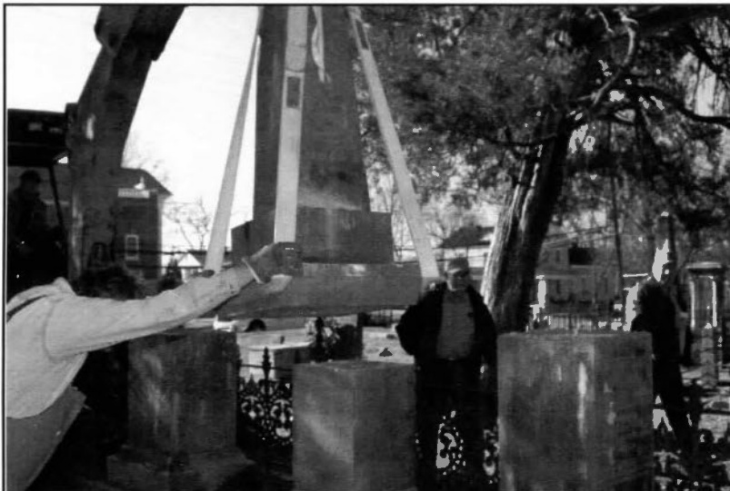
Two straps are used in a basket hitch to transfer the obelisk to the base. Note the 3" straps, each with an orange identification tag that lists the rated capacity of the straps under different conditions.
