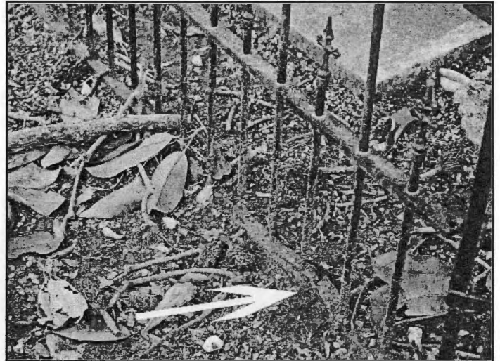
This photo shows the bottom rail and pickets buried in the soil. The arrow points out where the bottom rail has corroded away because of the ground contact. The ground level here needs to be lowered by about 6 inches.
