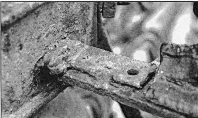
Here is an example of an inappropriate repair that detracts from the beauty of the fence and promotes additional damage. Spot welds allow moisture to migrate between the metal and cause additional corrosion.
