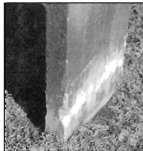
This stone shows the damage caused by improper use of nylon trimmers. The line is so heavy and the trimmer is use so close to the stone, that the marble is being cut away.
