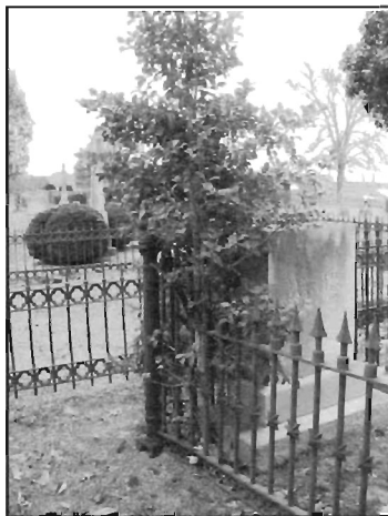
This tree has not yet caused irreparable damage and could be easily removed.
